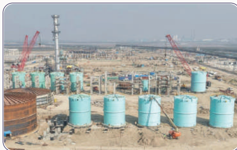
Largest FRP Site Fabrication Project in India. 10 nos. 500m 3 Storage Tanks. Project Location: Mundra, India
